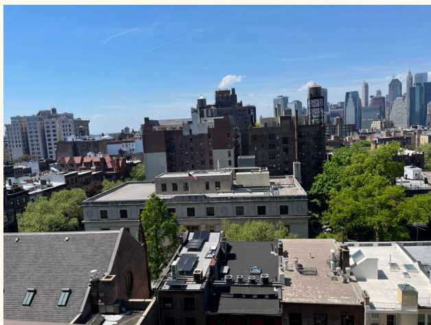
Rooftop solar array in Brooklyn. Photo: © Benjamin Spier
